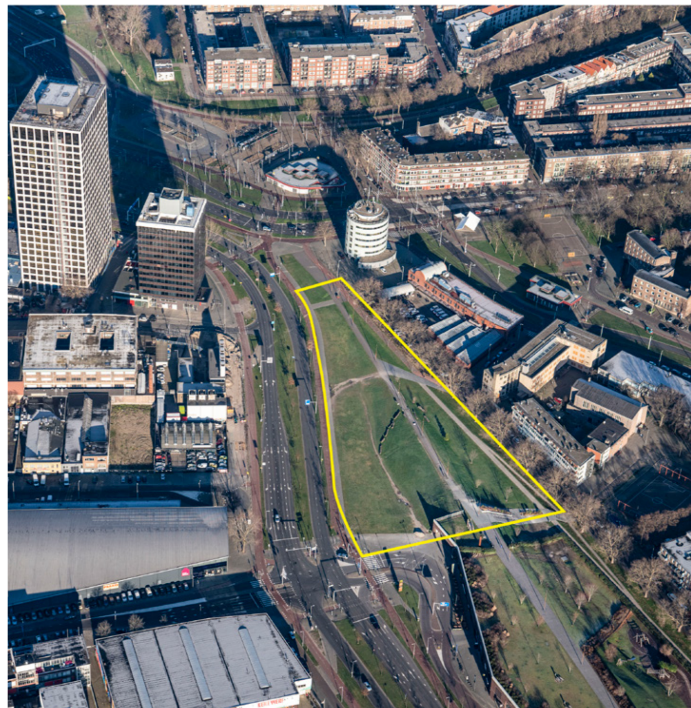
Kop Dakpark: project site (yellow)
