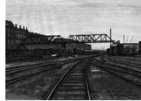
The pedestrian bridge provided dock workers from Bospolder with access to the port area
